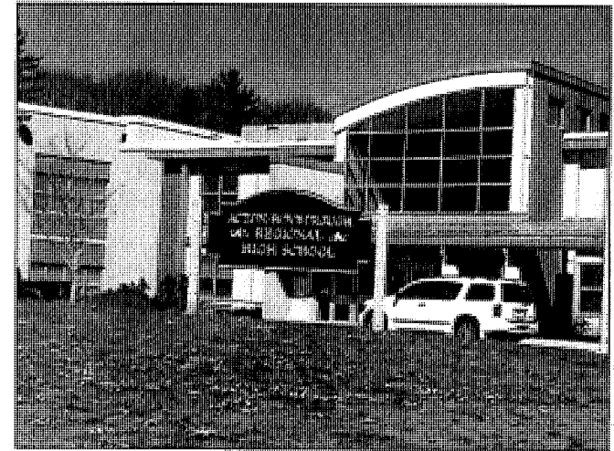
Acton-Boxborough Regional High School. WICKED LOCAL PHOTO/BILL FONDA
